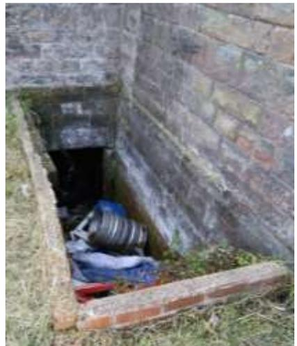
Underground plant rooms and their access stairways pose a number of hazards. Most in the author's experience are poorly-maintained with uneven, slippery steps and inadequate (if any) handrails. There should be a wall or railings around the opening to prevent anyone from falling in, with a padlocked gate to allow authorised personnel to access the plant room safely.
